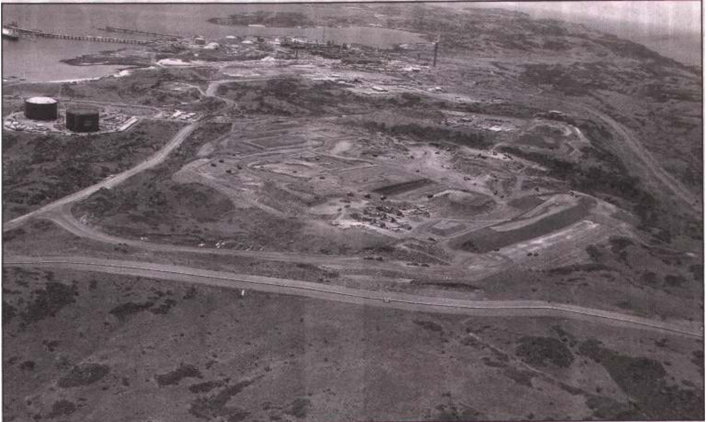
The aerial photograph taken by FARA, showing the Woodside Pluto development of its on-shore gas processing facility on the Burrup Peninsula in the Pilbara region of Western Australia.
