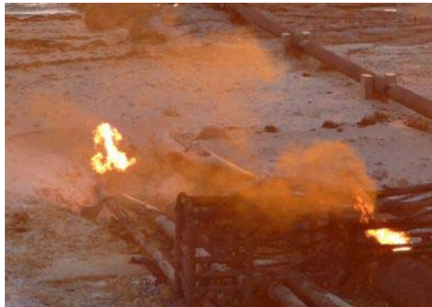
Fire damaged pipelines at Apache Energy's Varanus Island gas processing plant
