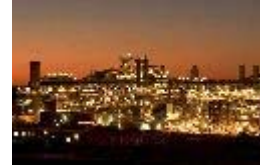
The North West Shelf onshore gas plant at Karratha
