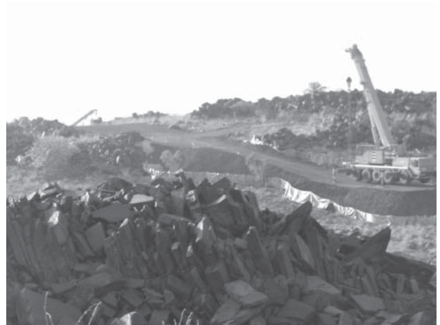
Figure 3. The mobile cranes move into position at Site A.
